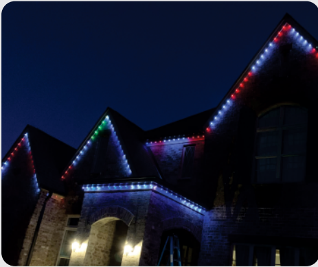
Lights seem to produce incorrect colors in the pattern or in certain sections.
